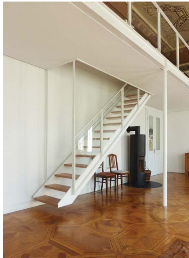
the stairs are suspended to keep the parquetry untouched
