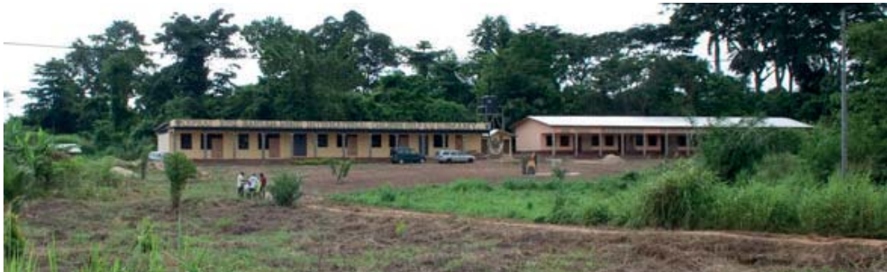
Site with buildings of first phase
