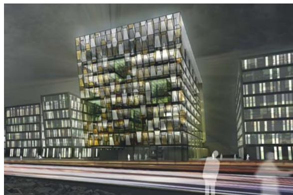
night view: headquarters addressing the prominent highway Sæbraut
